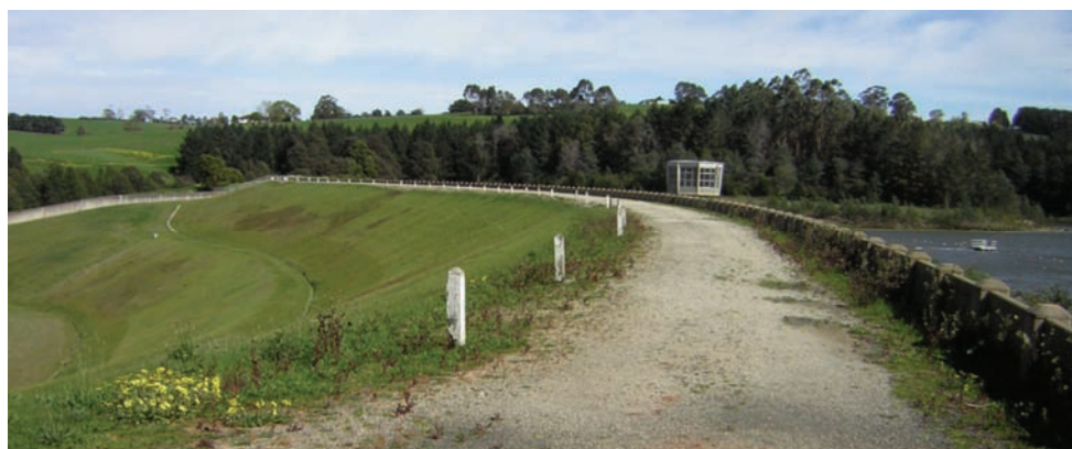
Tarago Reservoir, September 2009.
