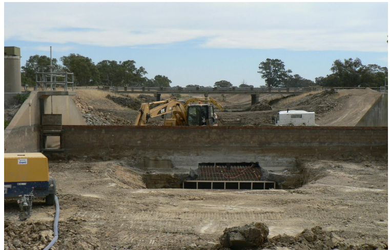
Above: Construction of drainage works for pump station Below: Outlet Channel deepening works in progress with construction of a hole below the flow measuring weir to allow water to pass up the channel to the new pump station.
