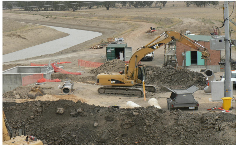
Above: Construction of drainage works for pump station Below: Outlet Channel deepening works in progress with construction of a hole below the flow measuring weir to allow water to pass up the channel to the new pump station.
