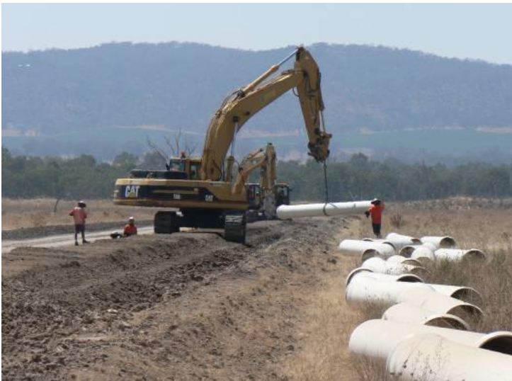
Laying of 450 mm diameter PVC pipe lengths in progress.
