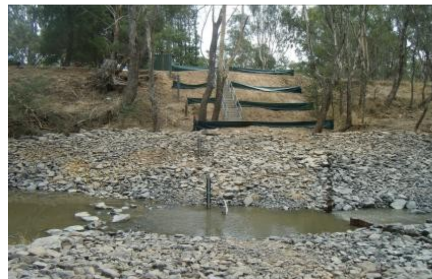
Figure 4: shows the upgraded low flow monitoring site at the Broken River At Orrvale, with new access steps, bank erosion controls, bank stabilisation and defined measuring point (sheet piling).
