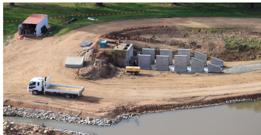
Fig 1: Broken River Bypass structure remodelling works
