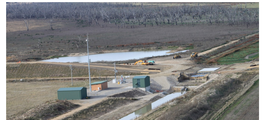
Fig 2: Embankment breach and pump station (foreground) with Winton Wetlands in background
