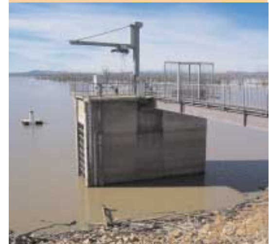
Mokoan Outlet Tower
