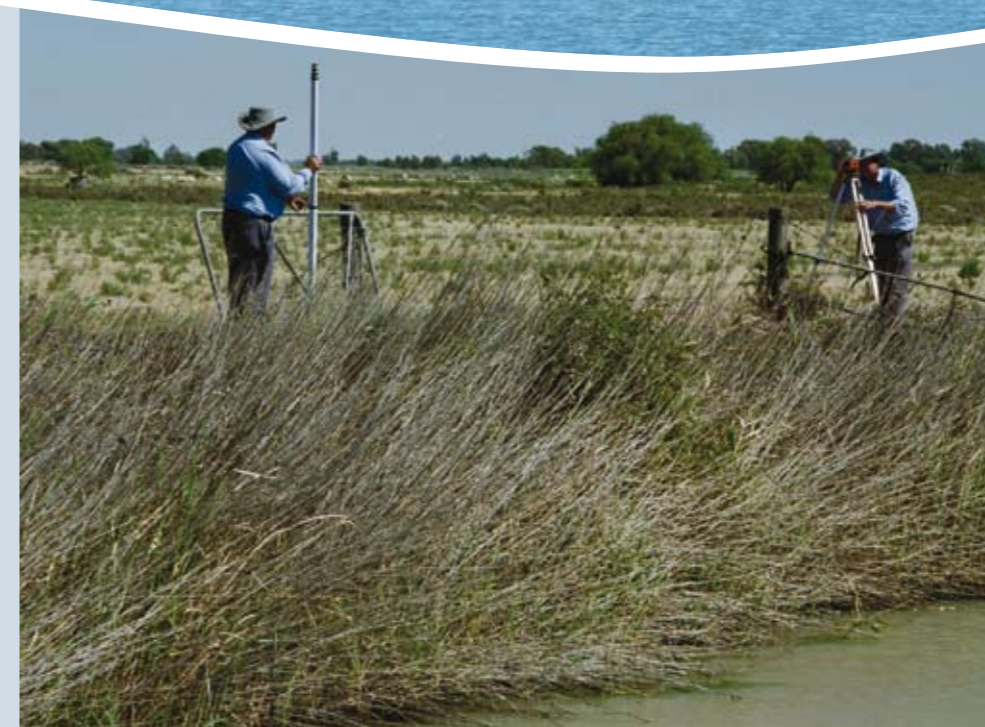
Goulburn-Murray Water staff surveying channel bank at Lake Boga. Photo courtesy of Tom Lowe
